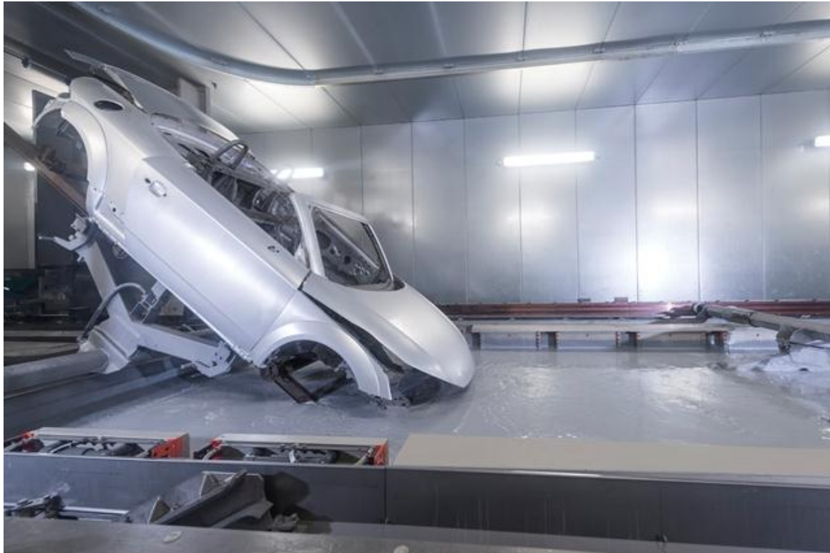
Fig. 3: In the splash-guard area, SCUBA moisture-proof luminaires were installed.
