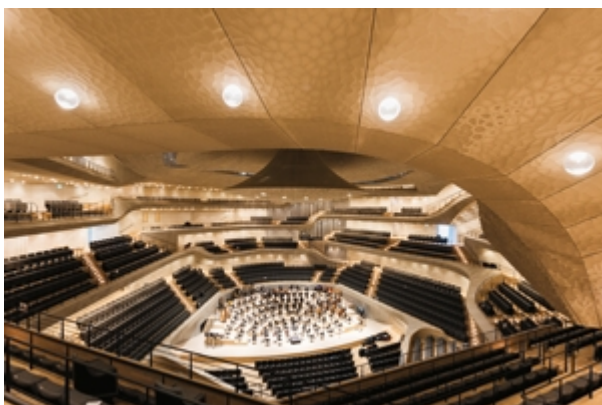
Photo 2: Zumtobel worked with Herzog & de Meuron and the glass designer Detlef Tanz from Wegberg to carefully craft 1200 hand-blown glass ball luminaires, which emerge from the undulating acoustic ceiling like light-filled water bubbles.
