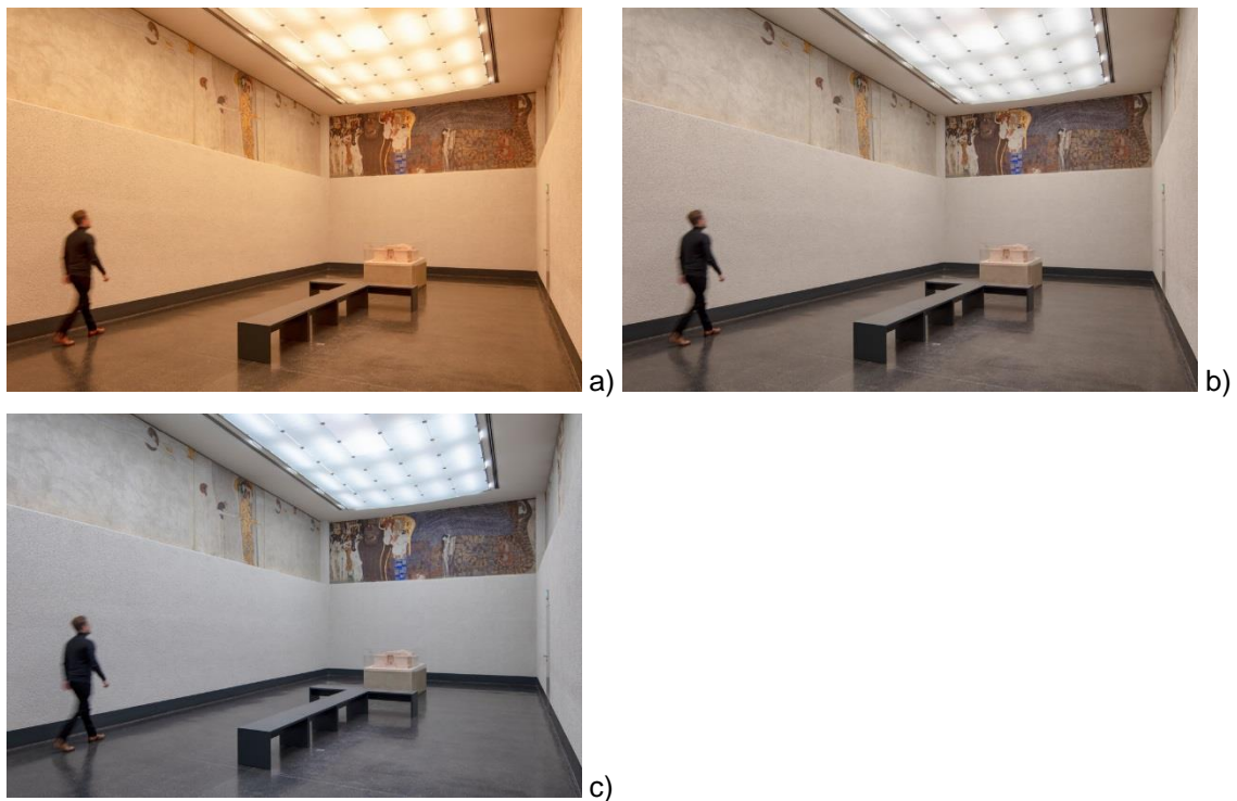
Fig. 3: While TECTON slim tunableWhite LED luminaires emit light for the ceiling in e.g. 3000 K (a), 4000 K (b), 6000 K (c), SUPERSYSTEM II LED spotlights immerse the Beethoven Frieze for the first time ever in direct wide-area light, creating an almost three-dimensional effect.
